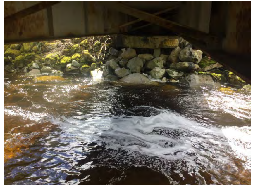
Right Bank Abutment when facing downstream
