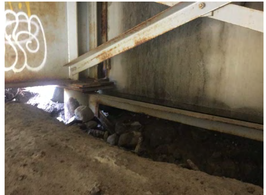
Right Bank Abutment when facing downstream
