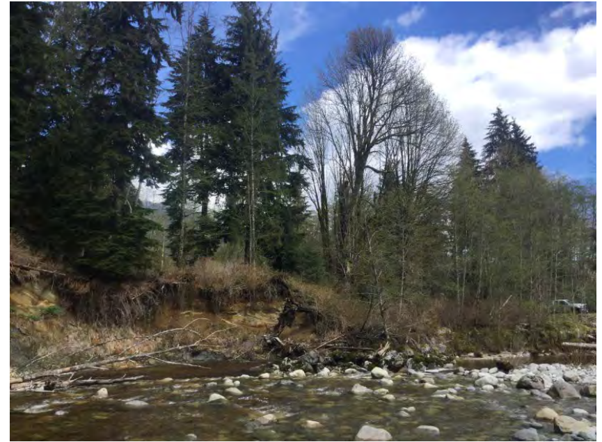
Upstream from Crossing - left bank upstream from crossing
