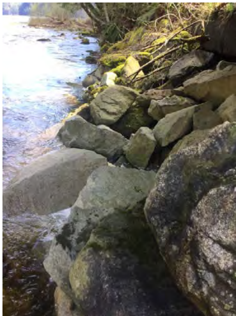
Right Bank Abutment when facing downstream
