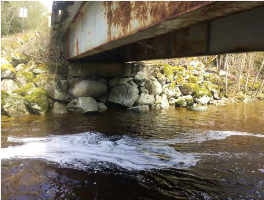
Left Bank Abutment when facing downstream
